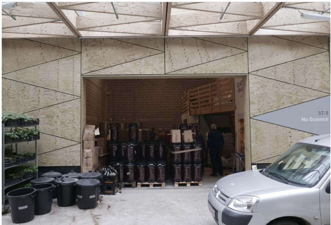
Greenbizz's productive groundfloor. The office spaces are located above. © Adrian Hill
